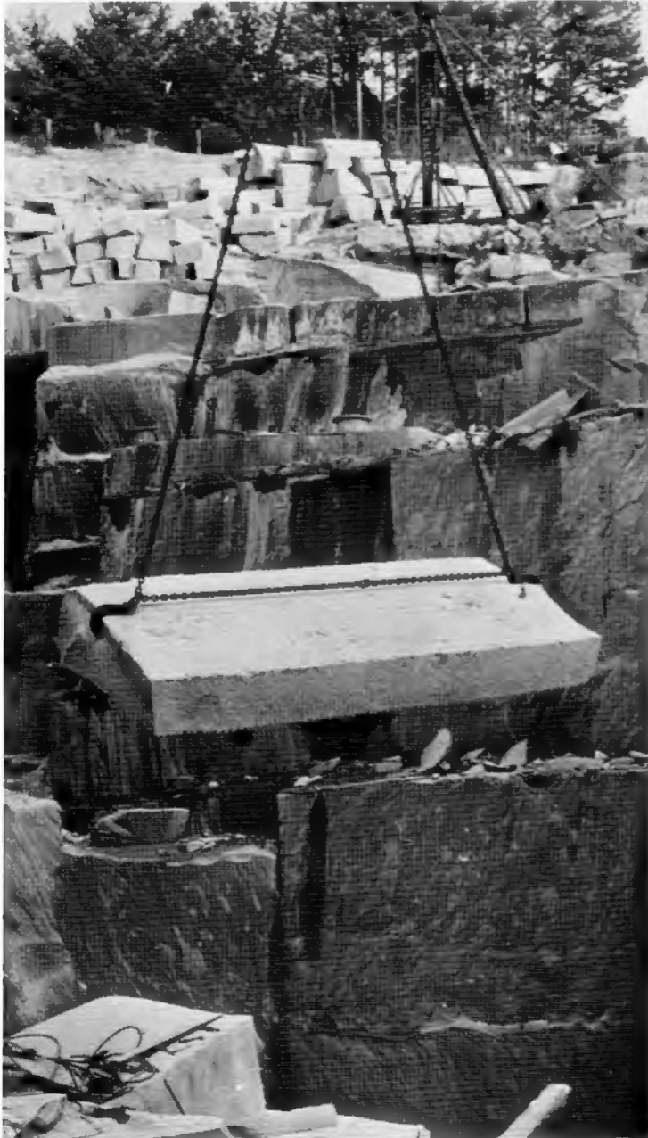
The first of The Georgia Guidestones ® blocks is lifted some 114 feet from the depths of Pyramid Quarry. Each block weighed approximately 26 tons.
